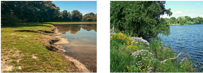
Figure 16: Eroded Shoreline Source: Dragonfly Pond Works versus a Natural Shoreline Source: VLAWMO
